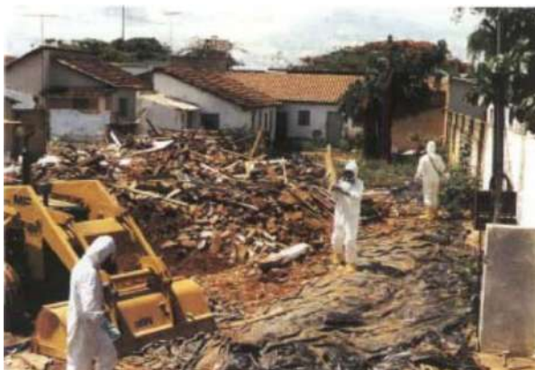
Figure 12. Demolition and Decontamination of the Scrap Dealer's House.
